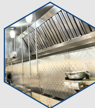
Kitchen Control Ventilation System
